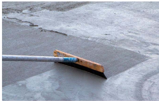
Figure 16: Brush texture on concrete
