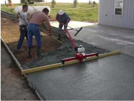
Figure 5: Vibrating screed
