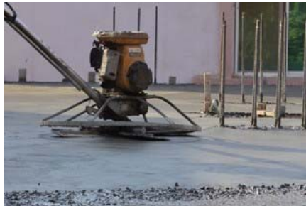
Figure 7: Vibrating Float
