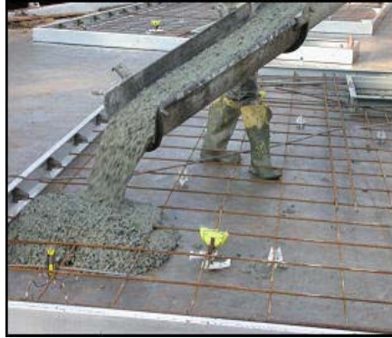
Figure 1: Reasonable slump concrete being placed near its final location.
