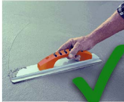
Figure 15: Magnesium float
