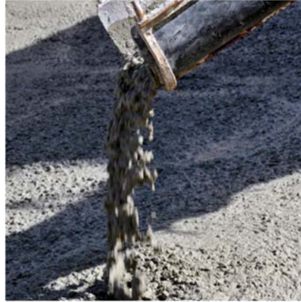
Figure 2: Concrete with excessive water creating high slump
