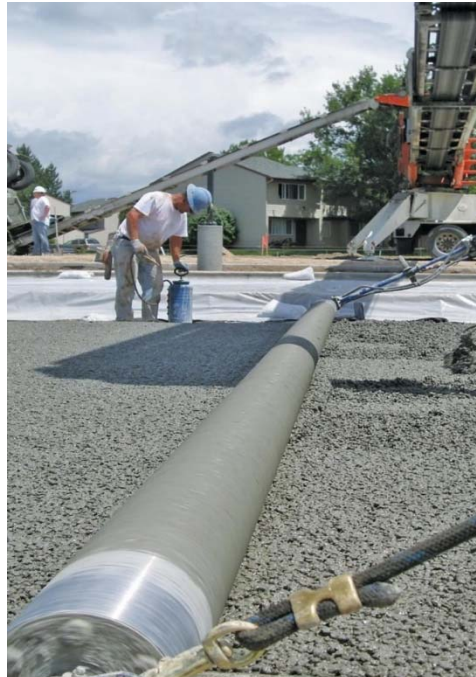
Figure 9: Roller screed
