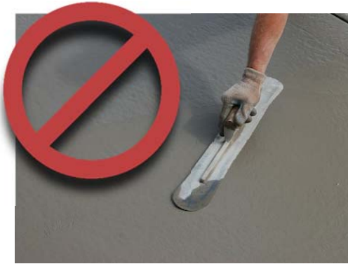
Figure 14: Steel trowel
