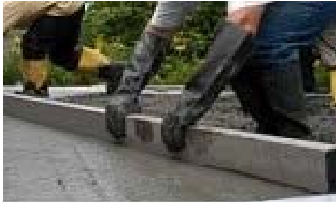
Figure 10: Metal straightedge
