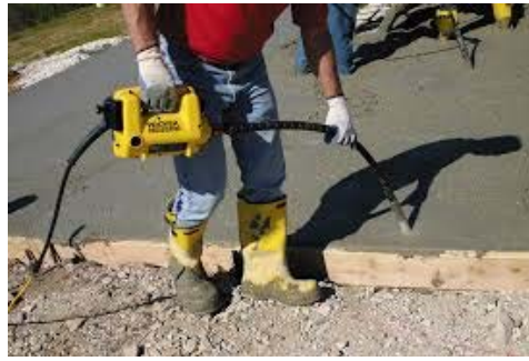
Figure 6: Internal vibrator
