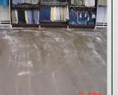
PROBABLE CAUSE 2 – Incompatible sealers have been used, causing trapped solvents between sealer layers
