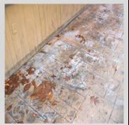
PROBABLE CAUSE 3 – A water based acrylic has been used that was either not mixed or applied too heavily.
