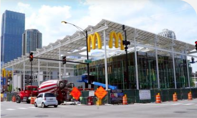
Chicago, IL - McDonald's Flagship Concrete Producer: Ozinga CO 2 Saved: 13.6 tonnes
