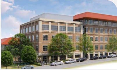
Austin, TX – UT Seay Expansion Concrete Producer: Lauren Concrete CO 2 Saved: 21.5 tonnes
