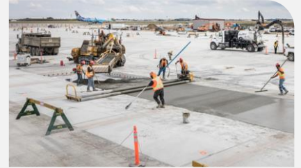
Calgary, AB – East Deicing Apron Owner: YYC Calgary International Airport CO 2 Saved: 160 tonnes
